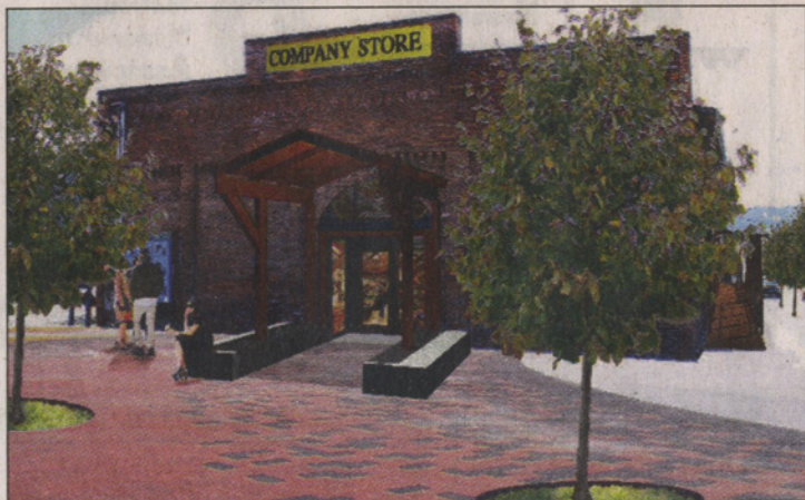
THE PROPOSED NORTH FAÇADE of the Roslyn NWI Building with the existing former loading dock door turned into a covered entry. The canopy is made from weathered steel and designed to compliment the industrial mining character of the building. Wooden entries to the building along the highway sides have been replaced with a hand-capped accessible steel porch and entry roof. Courtesy of Storefront Studio
